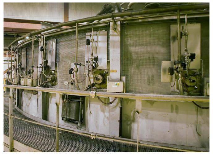
simple and compact oxyfuel installations at Ovako rotary hearth furnace
